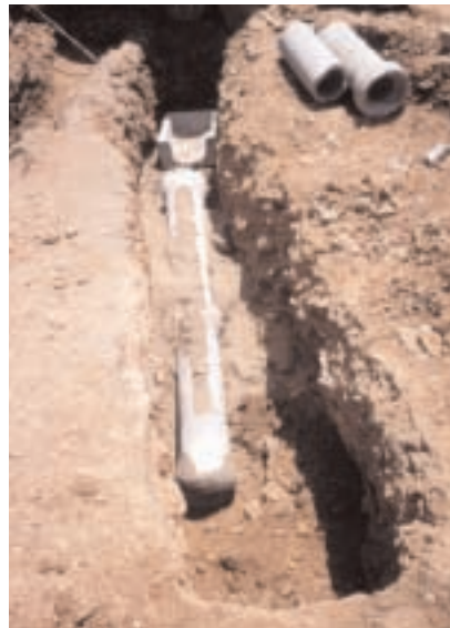
Fig. 2: A clandestine sewerage connection discovered while being made
