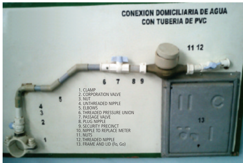
Figure 3. Drinking water connection scheme according to EPS internal regulations
