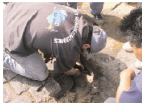
Figure 5. Clandestine connection cut
