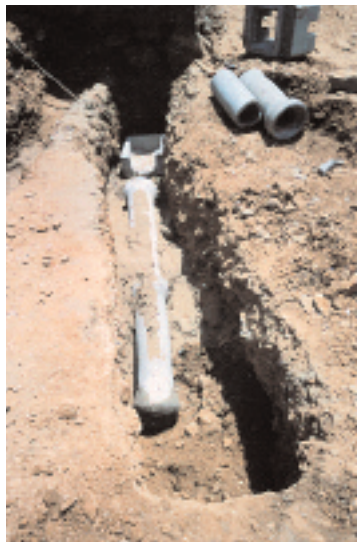
Figure 12. A clandestine sewerage connection found while being installed.
