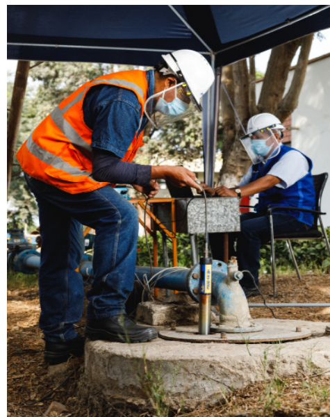
Groundwater monitoring with a probe at the water utility company Sedalib.
